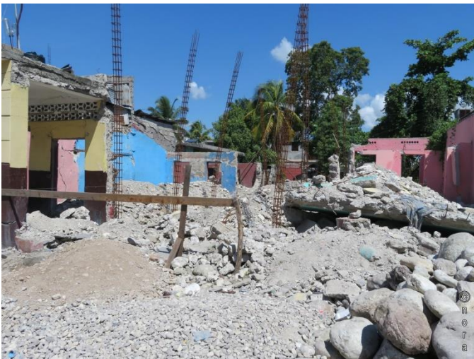
Homes lay in rubble and rebuilding efforts are slow to nonexistent.
