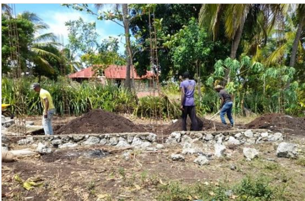
Foundation for Orphanage Kitchen
